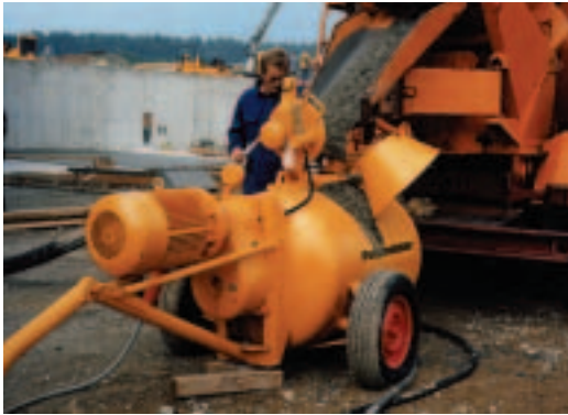
The M 500 E conveying floor-screed.
