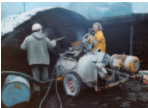
The M 500 E conveying earth-granulate.
